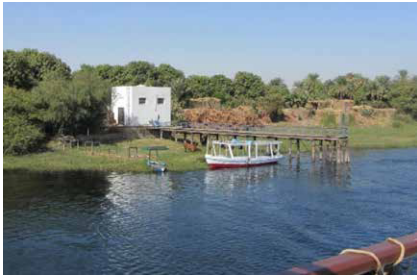
Fig. 7: Another pumping station along the Nile, which can be used for pumping bank filtrate
