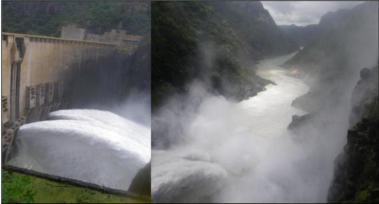
Figure 5.3: Cahora Bassa Dam April 29, 2010
