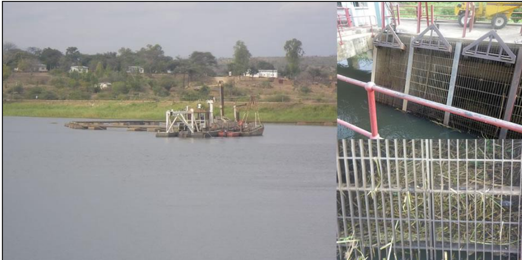
Figure 6.11: Trash management Nkula hydropower plant
