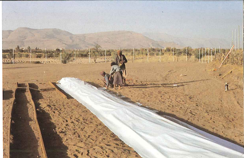
The supports are now covered with 0.1 mm plastic sheeting.
