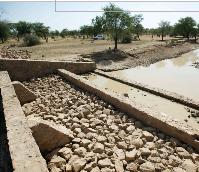
Water-spreading weir © GIZ / Klaus Wohlmann
