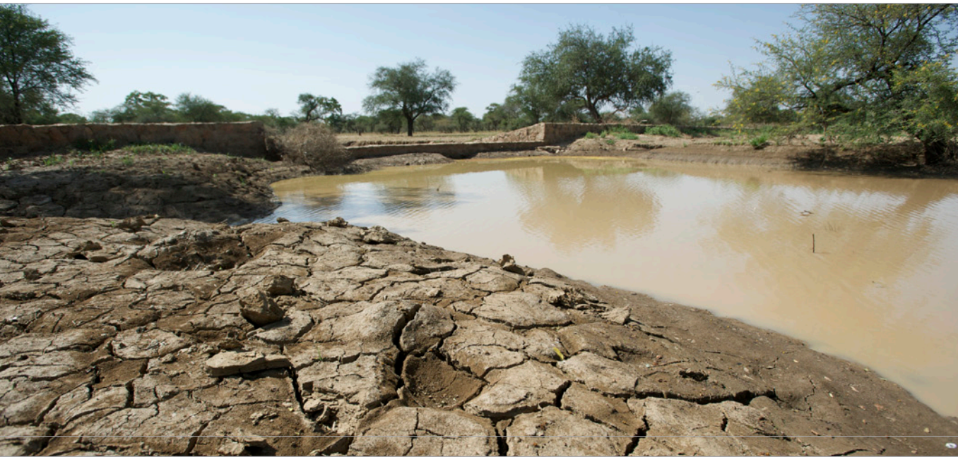
Water-spreading weir facilitates water supply and soil fertility © GIZ / Klaus Wohlmann
