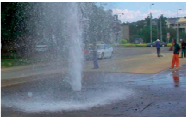
Pressure main bursts (USAID)
