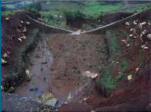
Figure 20. Arc-weir check dams constructed in big gullies
