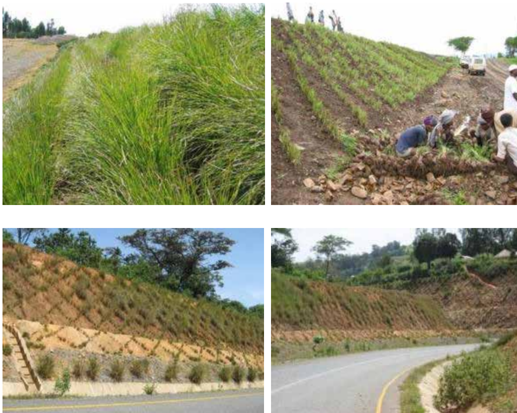
Figure 44. Bio-physical stabilisation of roadsides on the Bahir Dar–Gonder road (upper) and Assosa–Nekemte road (lower)
