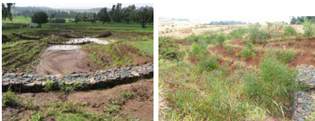
Figure 29. Gully sidewalls planted with grass and tree seedlings
