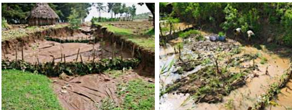
Figure 17. Reinforced bundling as an effective gully-rehabilitation measure
