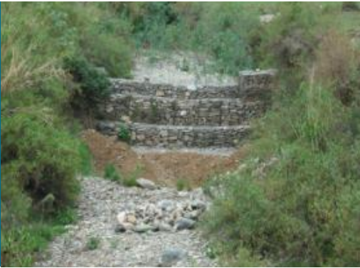
Figure 21. Gabion check dams as gully treatment
