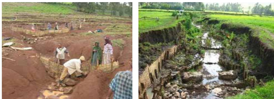
Figure 27. Bamboo and reed mats as gully treatment
