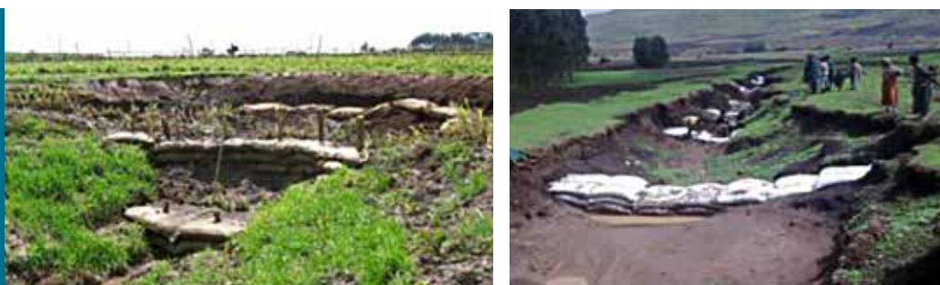
Figure 23. Sandbag check dams
