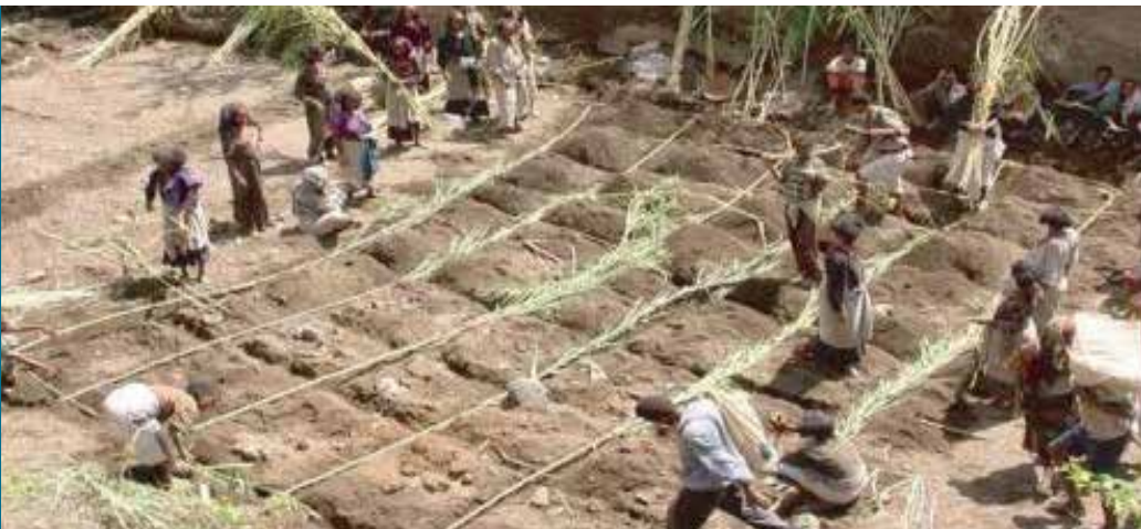
Figure 18. Treatment of degraded areas by layering vegetative materials – in this case, elephant grass
