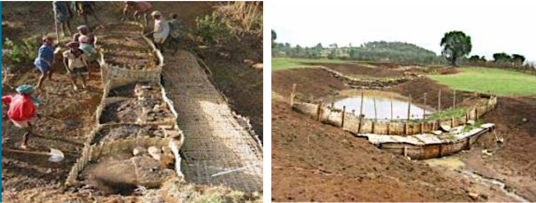
Figure 16. Organic bamboo gabion boxes and reed mats used in gully treatment
