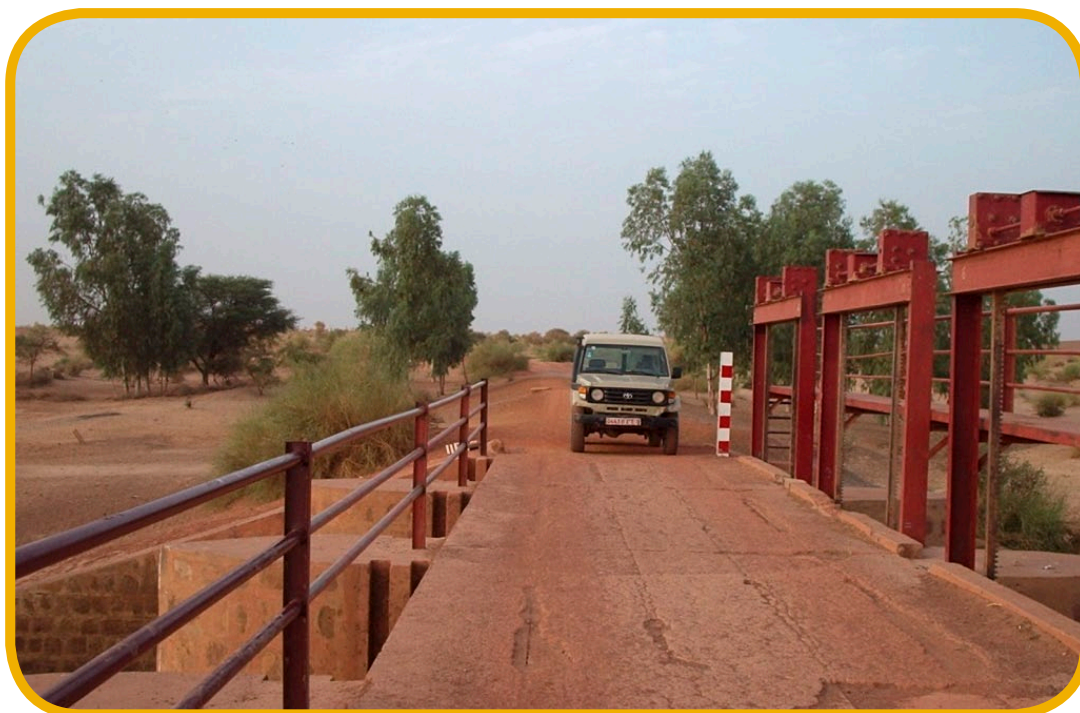
Photo 23 : Installation at Dabi on Lake Takadji
