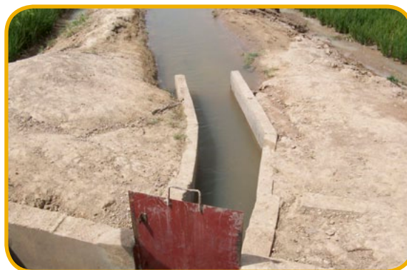
Photo 11: Turnout from a main canal into a secondary canal
