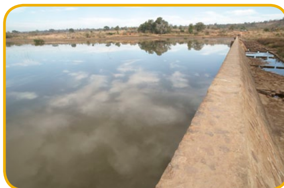
Photo 20 : Sounikéyni micro-dam in cyclopean concrete
