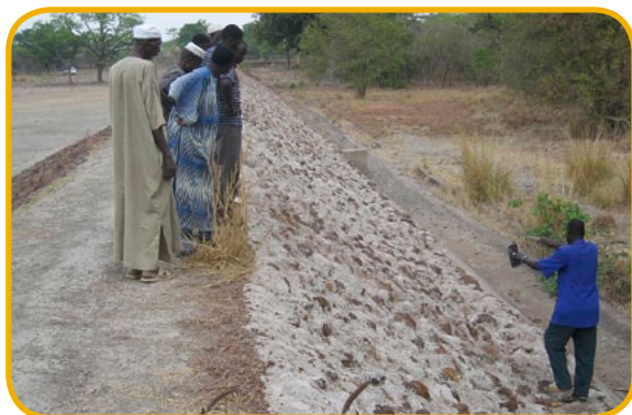
Photo 15: Earth embankment dam in Dioumantène (Kadiolo)
