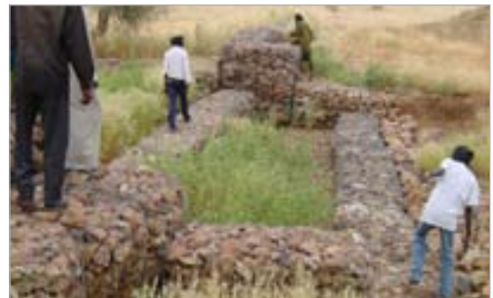
Spillway of a permeable rock dam with stilling basin. Source: PGRNG Mauritanie
