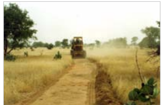
Creating a firebreak using a land grader.
