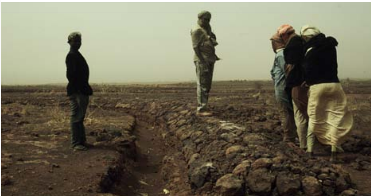
A contour bund inspected by engineers © GIZ / Martina Wegner
