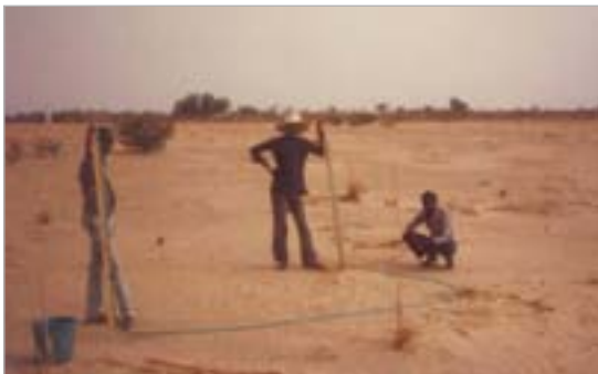
Water-tube level used to establish contour lines
