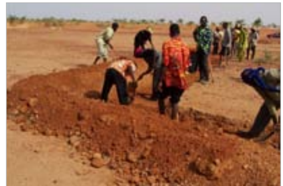
Construction of contour bunds. Source: CILSS
