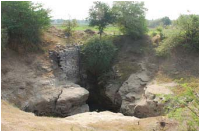
Wells in India must be dug deeper and deeper as the water table falls. This dry open well is a clear example of severe depletion of water tables.
