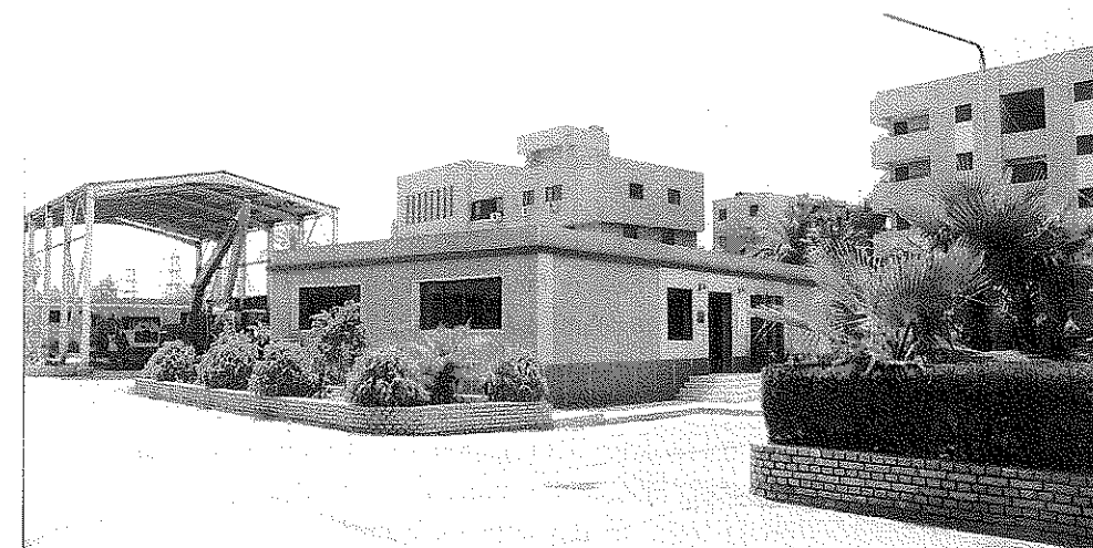
Drainage Training Centre—Tanta
