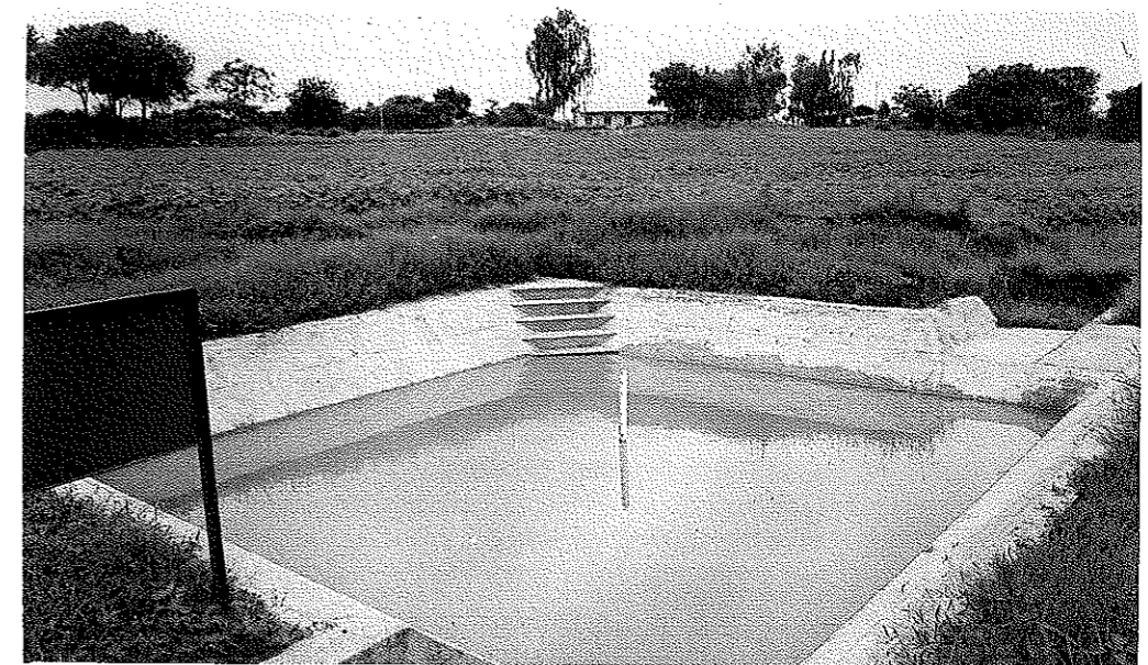
Water harvesting and recycling through dug out ponds: A key component of watershed technology
