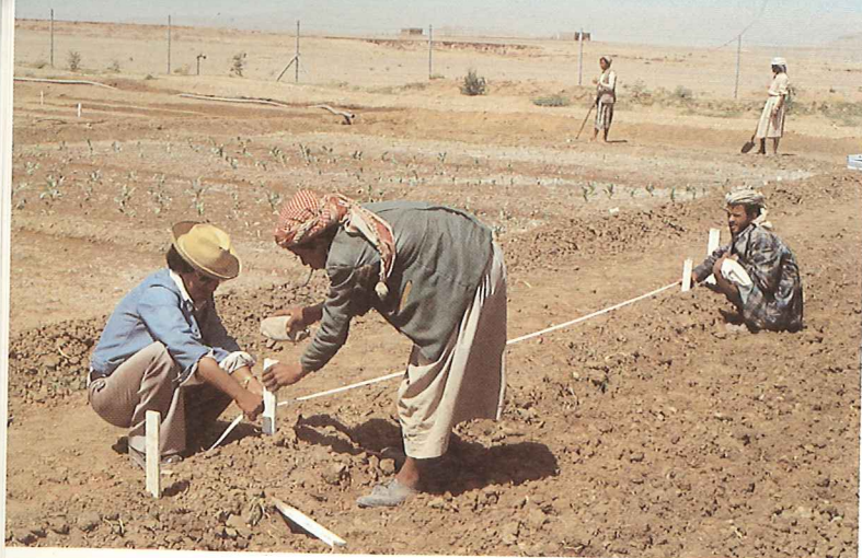
The distances of the basin ridges are measured and marked with pegs.
