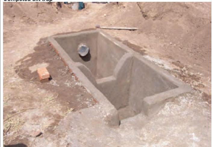
Completed silt trap
