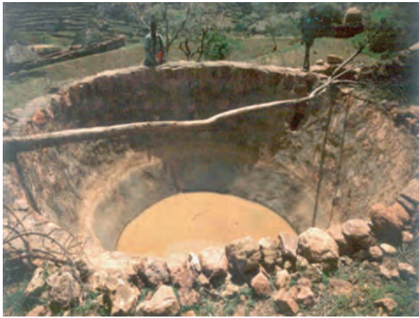
1. Illustration of cistern hemispherical shape - fig 1
