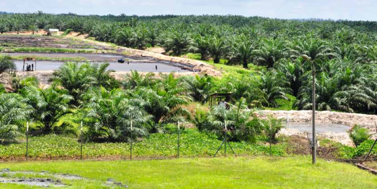
Stabilization pond of palm oil mill, Indonesia
