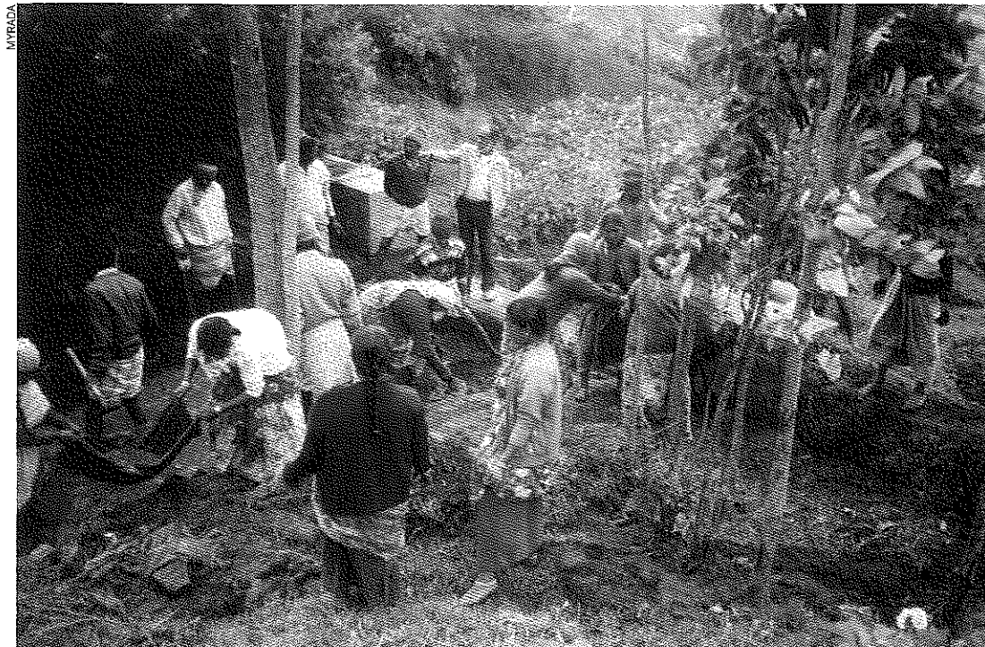
While it is important that this check dam be maintained, desilting has only occurred under the organisation and direction of outsiders (Katterry, T.N.)
